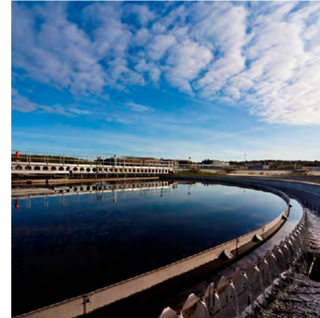
Spenn Valley Wastewater Treatment Works, Yorkshire, UK
