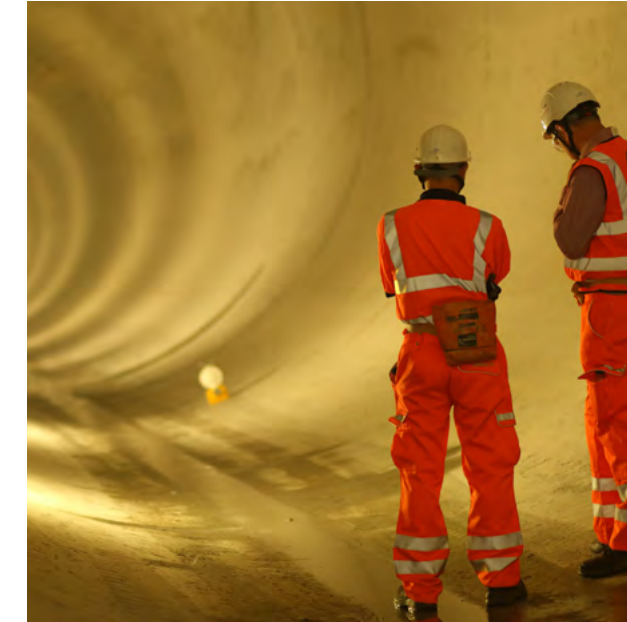
Lee Tunnel, London, UK
